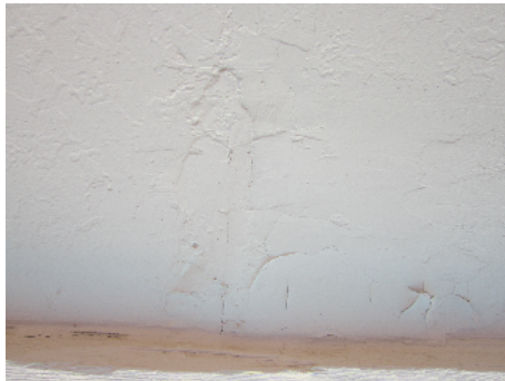
Minor patching to ceiling on patio, roof OK
