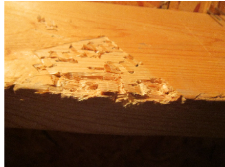
Truss nailing web observed in insulation and nailing web removed from upper truss member
