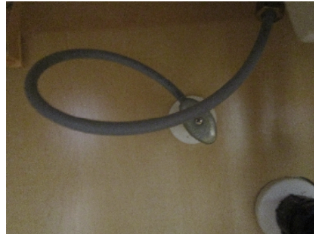
Upper Jack and Jill bath tub damage below water line older plastic supply lines and valves should be replaced
