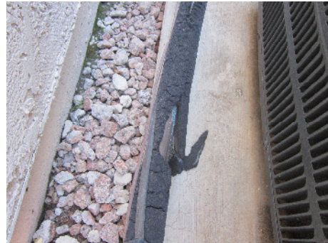
exterior AC coolant line insulation damage
