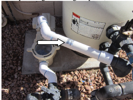
Pool plumbing PVC needs paint to prevent UV damage
