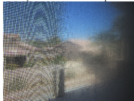
Lower hall bath window and upper master bedroom sliding glass door have lost seal
