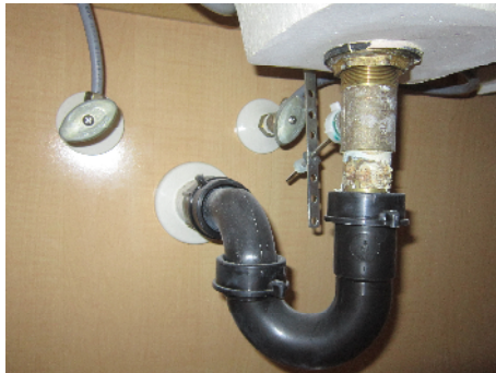
Faucet supply lines and stops old, tail pieces corroding minor water intrusion around windows
