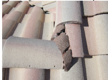
mortar caps broken need repair
