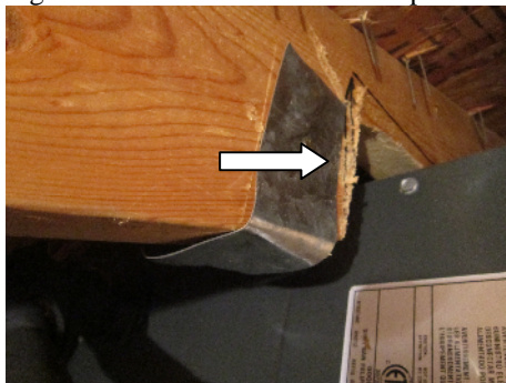
3 consecutive truss members were notched beyond 50% and a strut was removed during air handler installation
