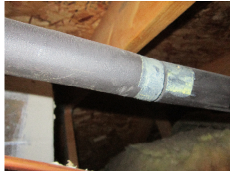
seams of suction line insulation need taping
