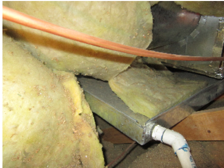
Duct insulation is laying in condensate pan
