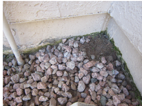
minor plumbing leak at rear foundation, possible pool filler
