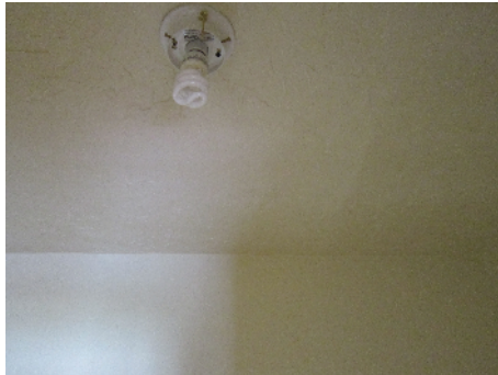
Drywall ceiling sagging from water damage in closet
