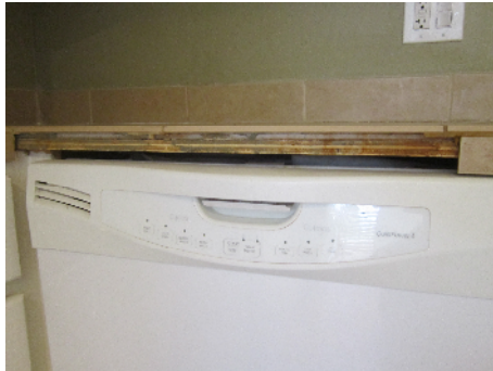
Damaged tile countertop in kitchen
