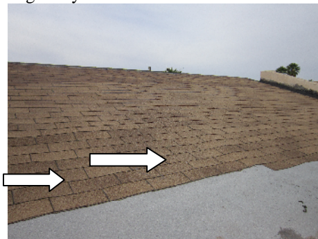
Ponding evidence on rolled roofing and seams patched sheathing sagging between rafters may be rotted
