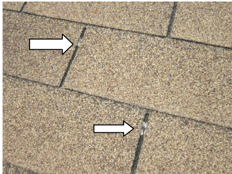
Roof shingles improperly nailed exposing many nails to water
