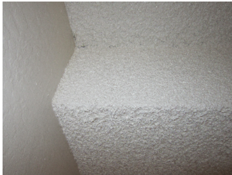
Possible asbestos in ceiling texture
