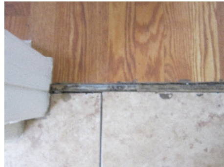
missing floor trim between tile and laminate
