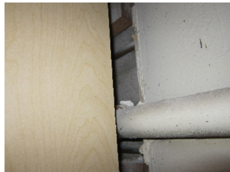
openings inside cabinets need sealing for insects
