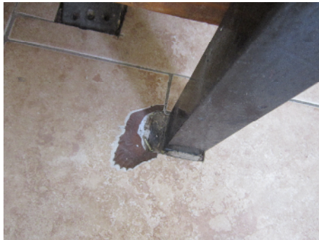
Loose stair railing and broken floor tile at stairway
