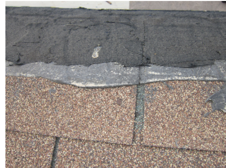
Roofing repairs recently done show cement patching only, no metal installed
