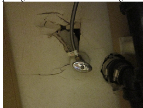
wall openings should be sealed for insects
