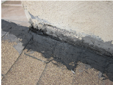
Roofing repairs recently done show cement patching only, no metal installed
