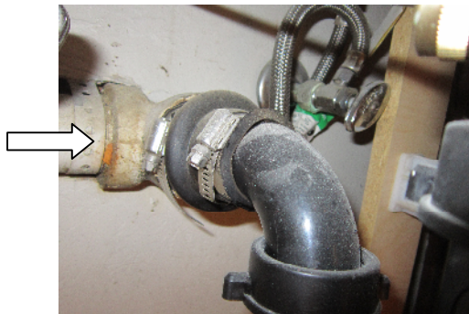
Drain pitch improper and connection suspect
