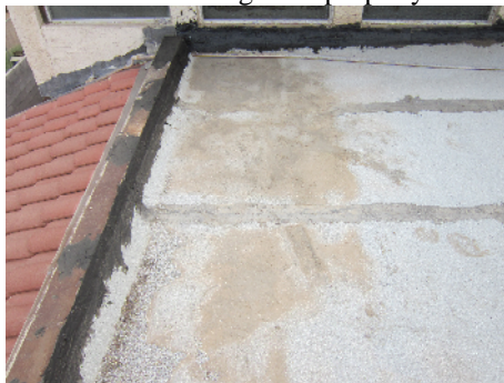
Ponding evidence on rolled roofing and seams patched sheathing sagging between rafters may be rotted
